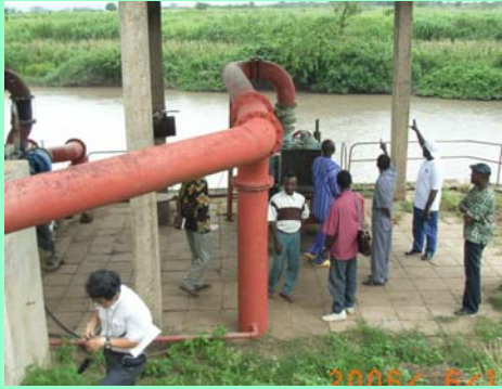
Water level of the Mono R. Is still too low for pumping-up
